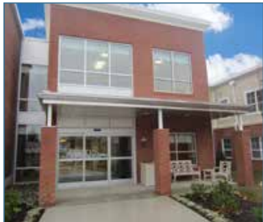
Springside School Senior Housing • Burlington Township, NJ NJ Future Smart Growth Award Architect: Kitchen & Associates
