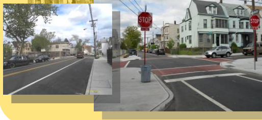
Streetscape work complete
